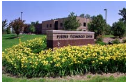
exterior Technology Center Download photo
